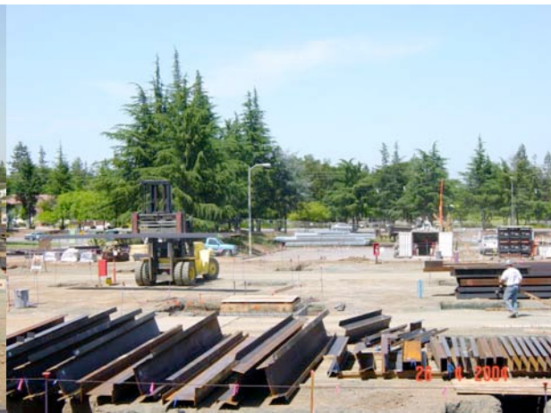
Maneuvering the steel supports
