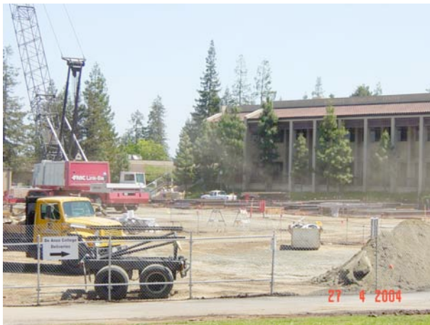
Looking south toward the ATC building
