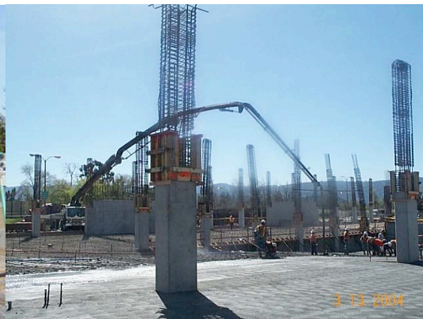
Pouring the concrete
