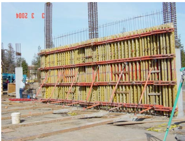
Building the shear walls
