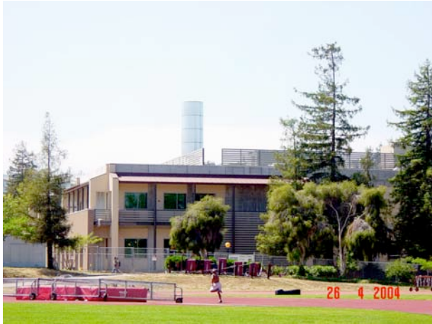
View of Lab Building looking West
