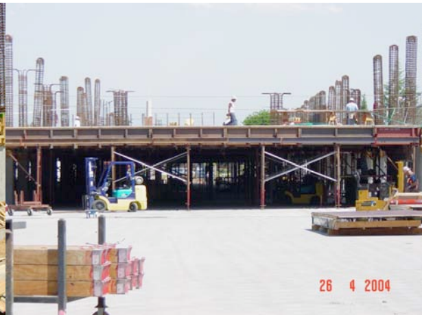
Erecting the second level
