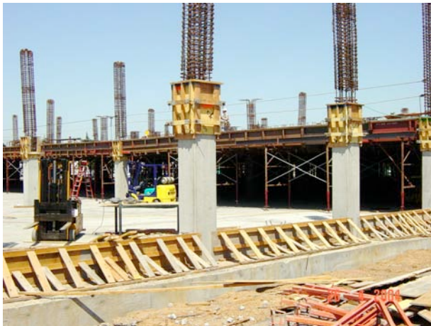
Erecting the second level
