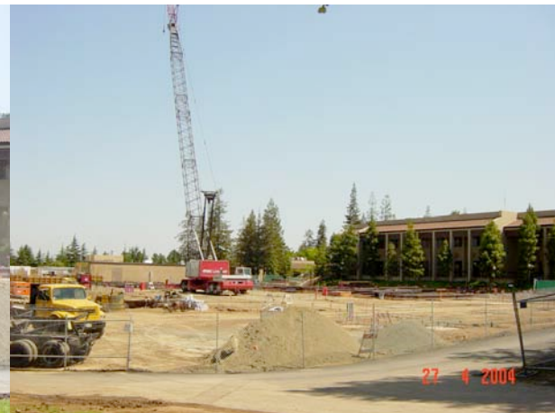
The crane arrives on campus
