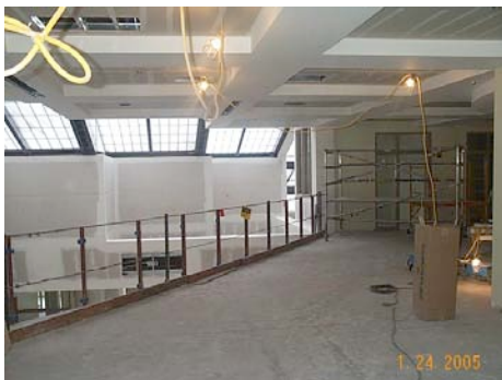
SCS Interior Upper Level
