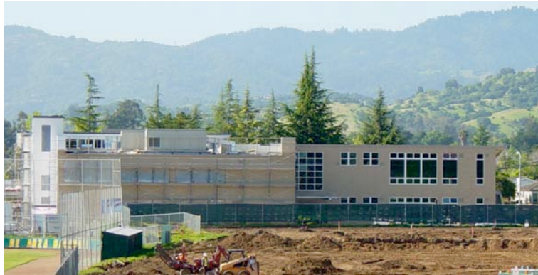
Kirsch Center Exterior North Facing
