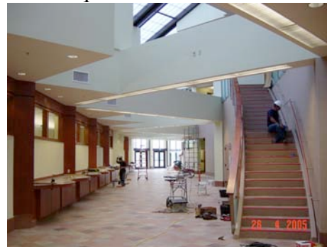
SCS - Main Lobby
