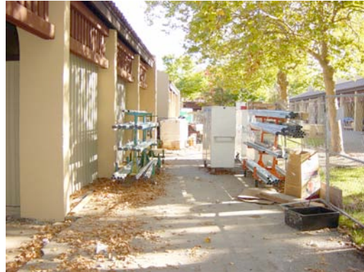
New Windows & Doors
